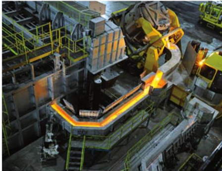
Vedanta has state-of-the-art PFA casting facilities in Chhattisgarh and Odisha producing ingots, billets, wire rods and rolled products.
